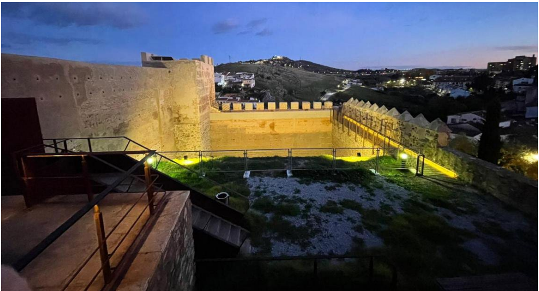
Baluarte de los Pozos, opened to the public in 2021 as part of the rehabilitation of Cáceres Walls project
