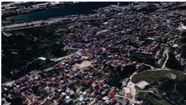
Illegal and unplanned private housing
