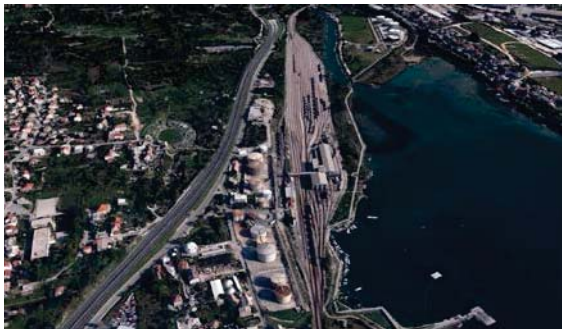
Industrial and infrastructural zone
