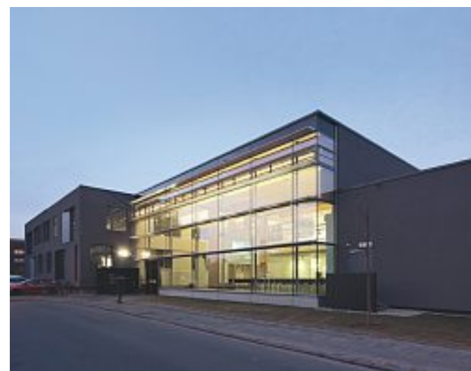
University of Applied Sciences, Darmstadt before and after retrofit 2010/11, Cornelsen and Seelinger Architekten
