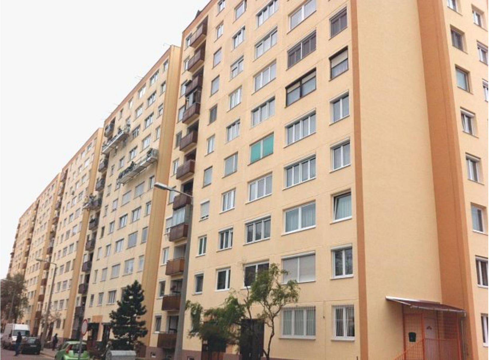
Retrofitting 315 flats in Budapest with new external wall insulation and solar heating
