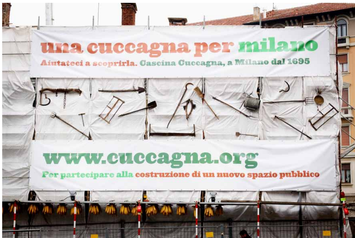
Cascina Cuccagna, during renovation 2009. Photo: Courtesy of Cascina Cuccagna
