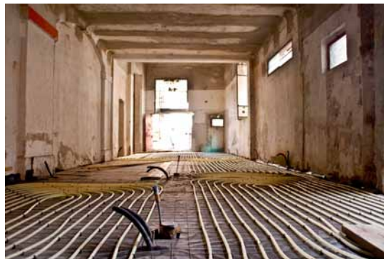
Cascina Cuccagna, geothermal pipes installation, 2009 Photo: Courtesy of Cascina Cuccagna
