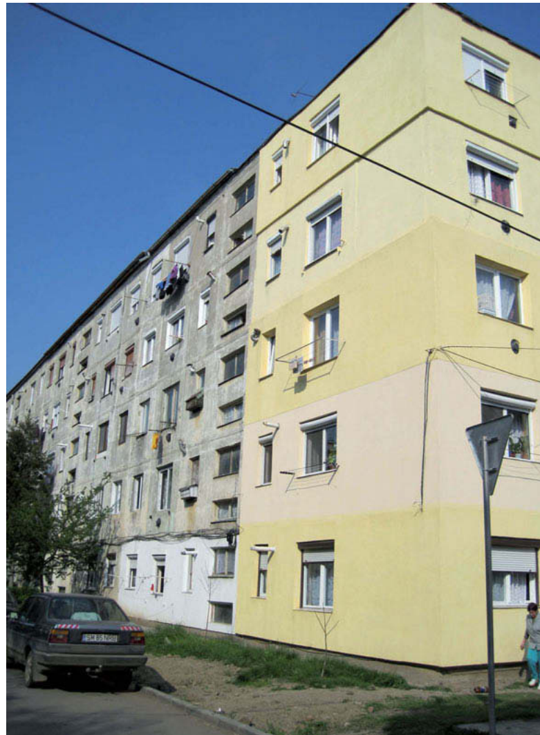
Privately owned apartment block with renovated facades in part of the apartments, Satu Mare
