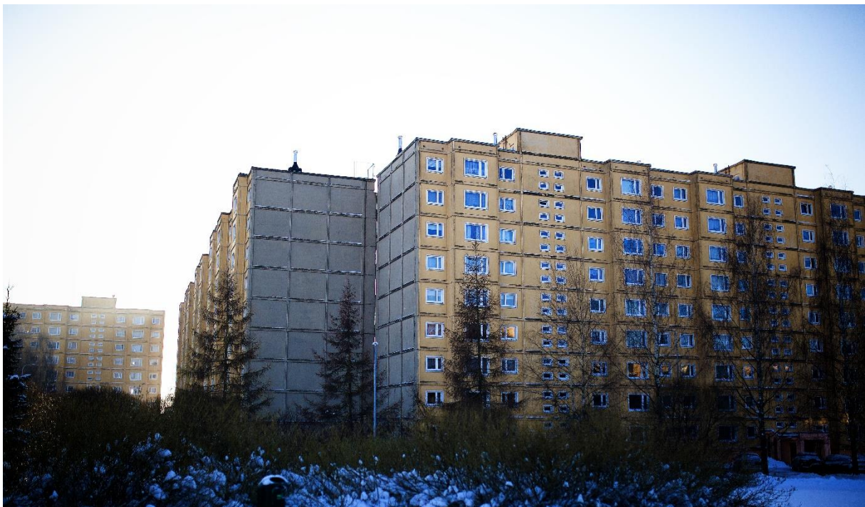
PHOTO6: ANNEMÕISA STREET APARTMENT BUILDINGS BY TIINA PITK
