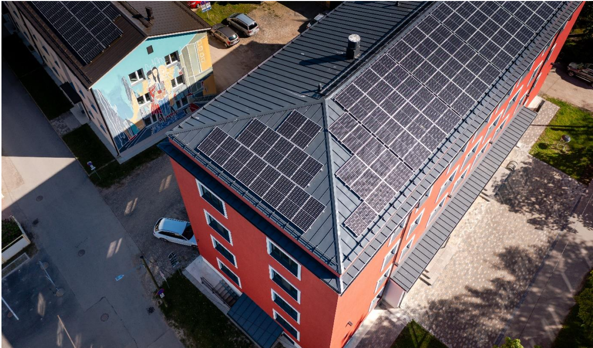
PHOTO4: NEWLY RENOVATED TIIGI 19 AND TIIGI 21 APARTMENT BUILDINGS WITH SOLAR PANELS BY SILVER SIILAK
