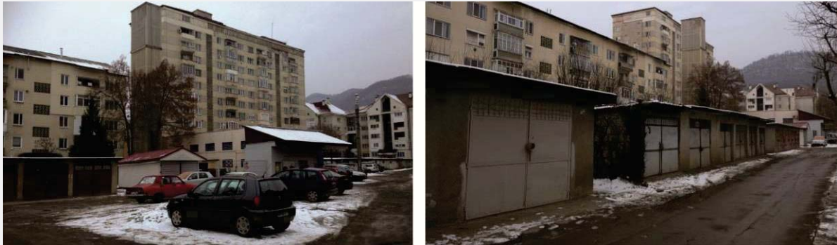
The pilot area (collective housing, and private garages/ indoor parking lots)
