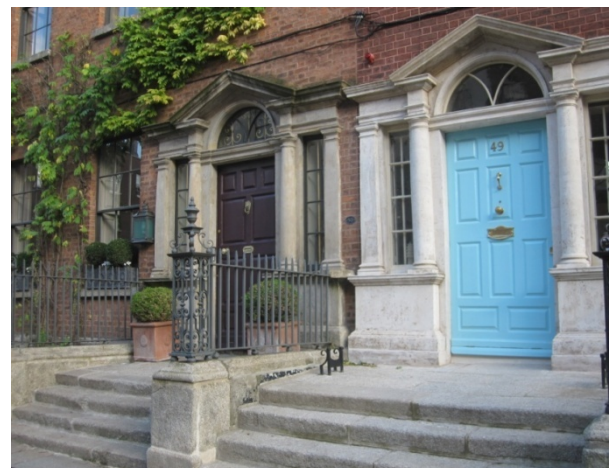
Figure 2.10: External steps of a Dublin Georgian Building
