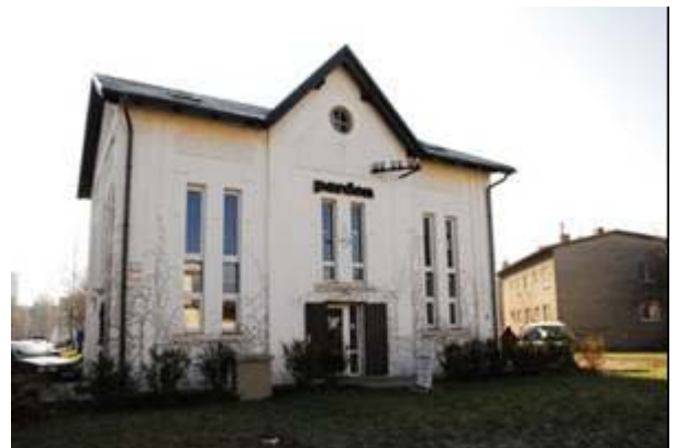
Figure 2.19: Trafostanica (Power Sub-Station) in Nitra
