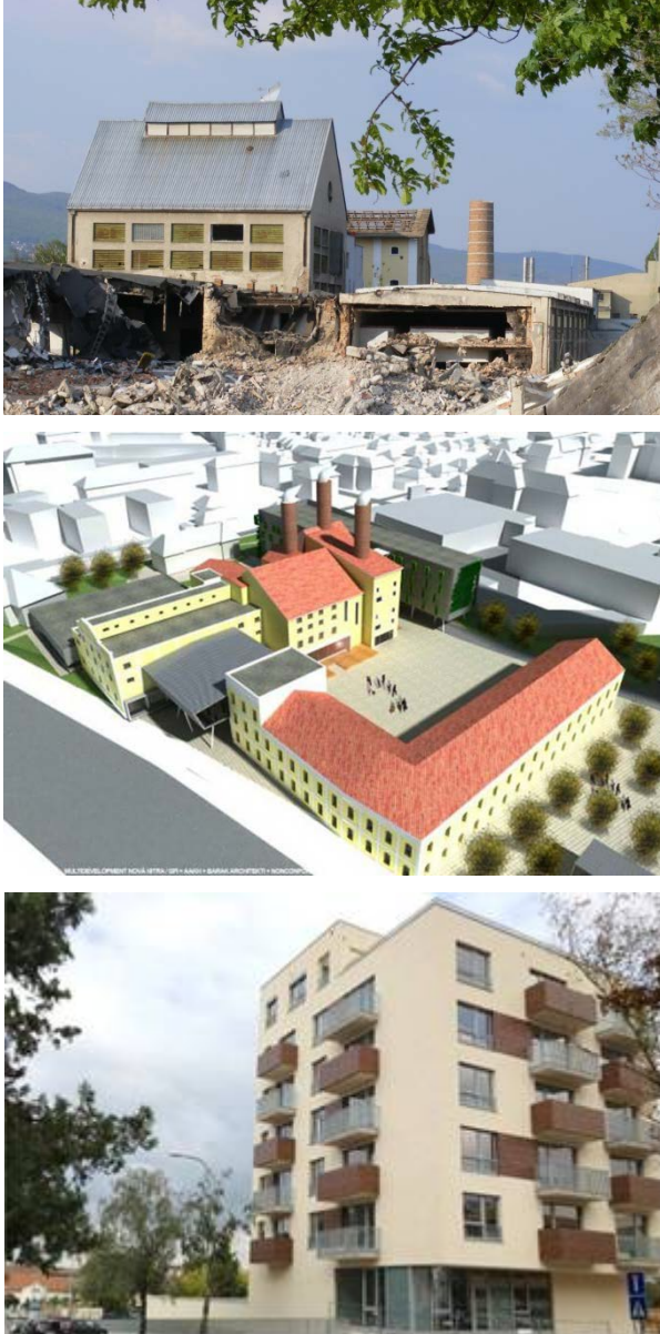
Figure: 2.20: Nitra – “City Brewery” redevelopment
