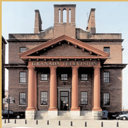
7. Albert Dock Traffic Office 1846-7 Grade I This is one of a number of building designs by Hartley in collaboration with Philip Hardwick. It is built of brick with red sandstone dressings. The most remarkable feature is the cast iron Tuscan portico and frieze. The building was restored with the rest of the Albert Dock by the Merseyside Development Corporation in the 1980s. It is now owned by National Museums Liverpool and will become home to the International Slavery Museum.
