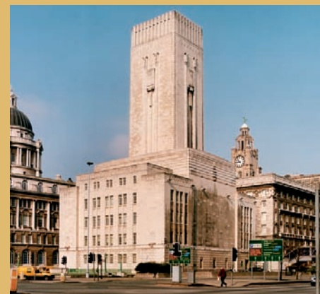
4. George's Dock Tunnel Ventilation Building and Offices 1931-1934 Grade II This stylized obelisk, reminiscent of ancient Egypt, was designed by Sir Basil Mott and J. A. Brodie, with Herbert J. Rowse, to serve the Mersey Road Tunnel. It has statues of Night and Day, symbols of the never-closing Mersey Tunnel and a black marble memorial to the workers who died in its construction.
