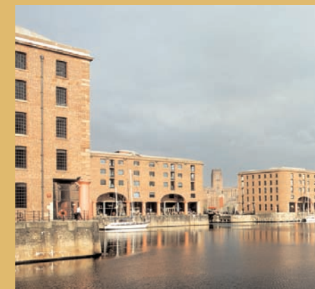
6. Albert Dock Warehouses Opened 1846/7 Grade I Opened 1846-47 Albert Dock Warehouses form the largest group of Grade I Listed Buildings in England. Jesse Hartley used well-established techniques adapted from textile mill methods. He introduced new solutions, such as the amazing stressed-skin iron roof. Raising of goods from the quaysides was performed with the first hydraulic cargo-handling installation in the world.
