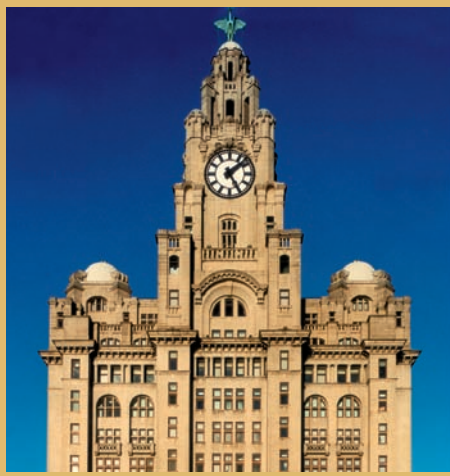
1. Liver Building 1908-11 Listed Grade I The head offices of the Royal Liver Friendly Society were designed by Aubrey Thomas. It is notable as one of Britain's first multi-storey reinforced concrete framed buildings. The clock towers are mounted with copper Liver Birds which to many are the very identity of Liverpool.
