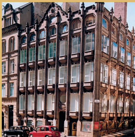
14. Oriel Chambers 1864 Grade I Designed by Peter Ellis, the use of oriel windows was driven by a desire to provide good daylight. The oriels themselves are framed in the thinnest sections of iron. In its day, the building aroused much opposition. It is only recently that its futuristic qualities have become appreciated.
