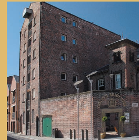
19. The Bridewell 1861 Grade II Located in the Duke Street area, the Bridewell, or Police Station, dates from c.1850. It is of brick with stone dressings and a slate roof. The building is of two storeys and three bays, with the centre bay projecting to form the base of a short tower. The Bridewell is now a public house and restaurant.
