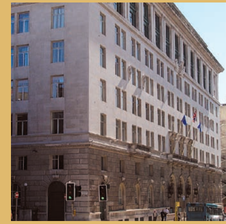
12. India Building 1924-31 Grade II This immense office block was built for the Blue Funnel Line and designed by Herbert J Rowse with Briggs, Wostenholme and Thorneley. It has stripped classical facades; Italian Renaissance detail is restricted to the top and bottom storeys. The building was badly damaged in the war, and restored under Rowse's supervision.
