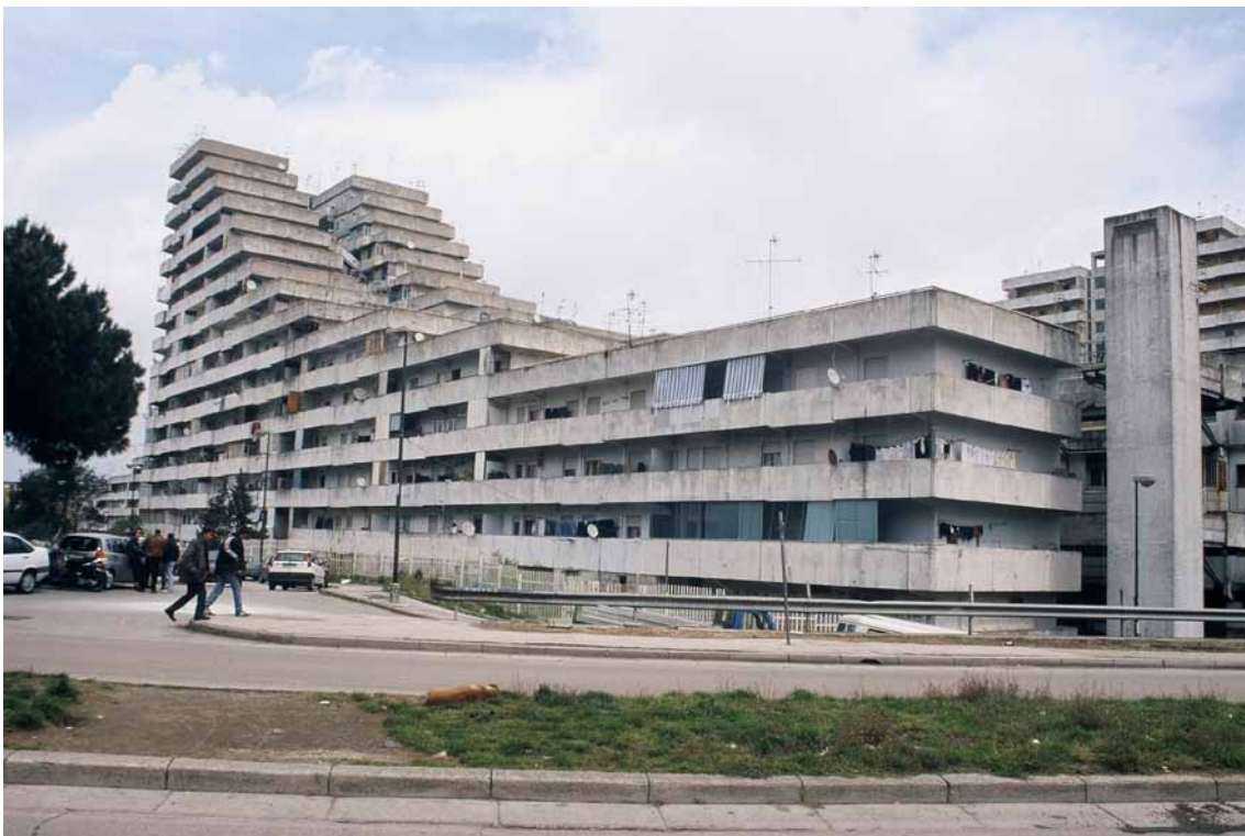
Naples, Scampia housing estate, one of the “famous” Vele buildings in 2003. Photo: Iván Tosics
