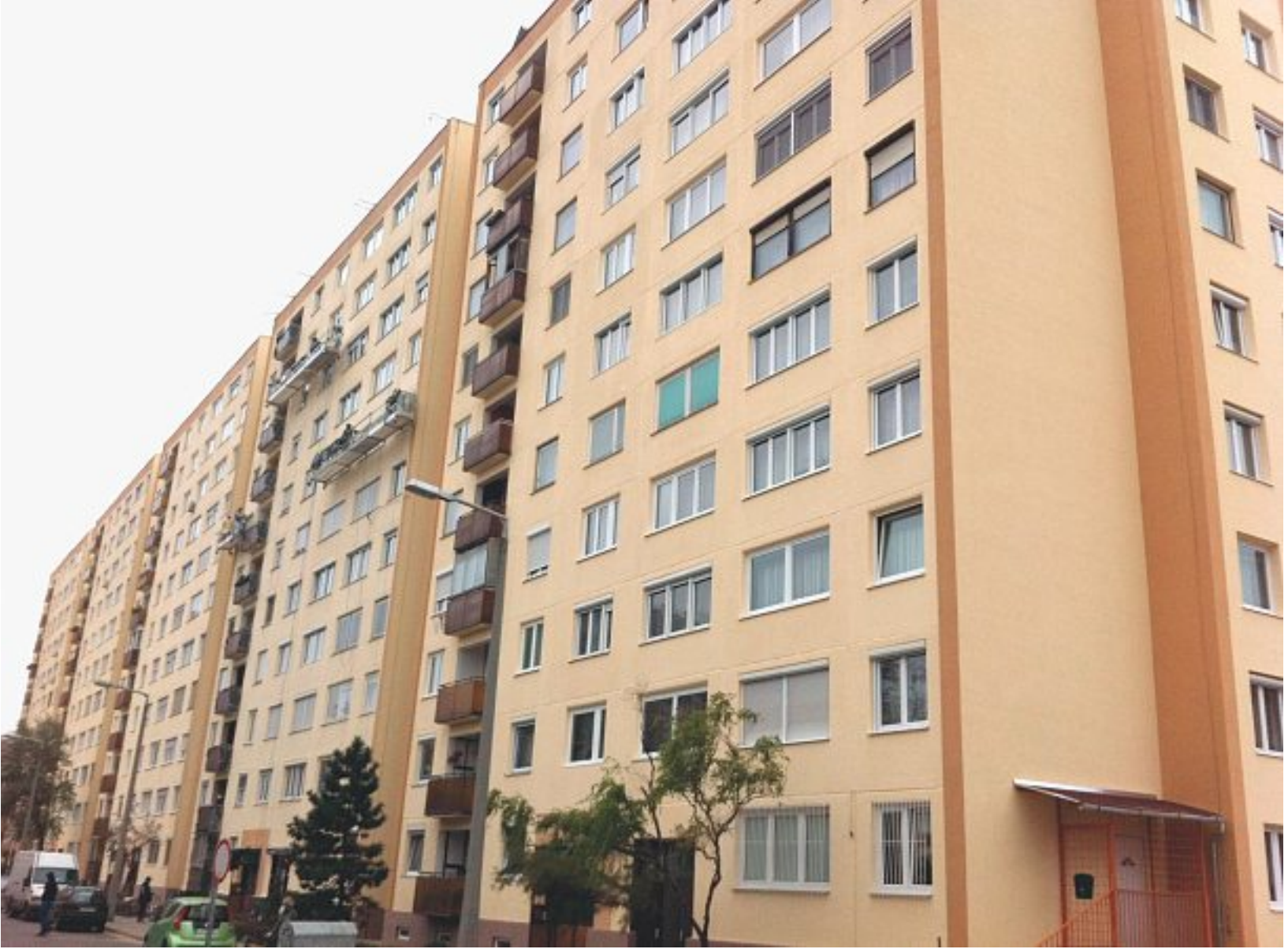
Retrofitting 315 flats in Budapest with new external wall insulation and solar heating
