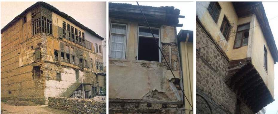
Fig. 11 Earth block buildings in Greece
