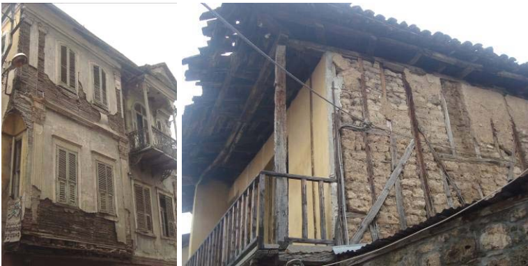
Fig. 1. Typical old structures in Veria
