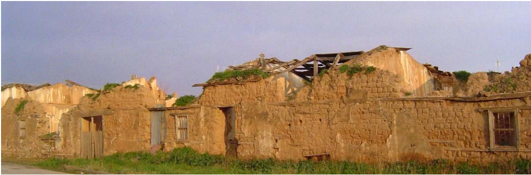
Fig. 20 Village Zografou Chalkidiki. Block of workers' houses (1845 A.C.)
