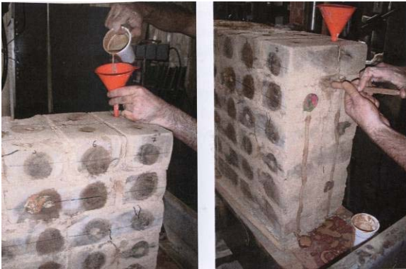
Fig. 18 Technique of grouting earth block masonry with soil based grouts
