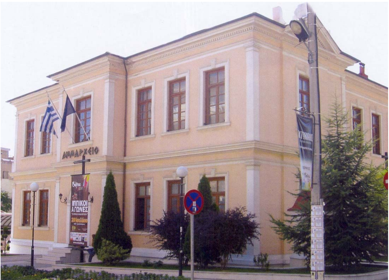
Figure 1. Town hall of Veria
