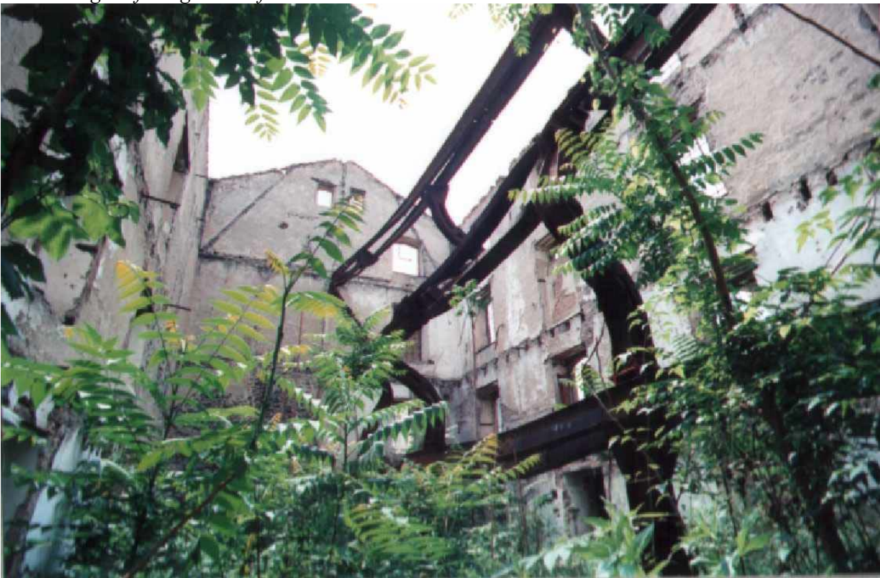
Figure 2. The internal space before the restoration works
