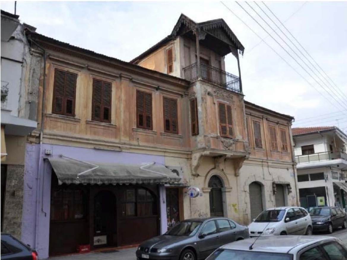
Figure 1: View of Chatzikou House
