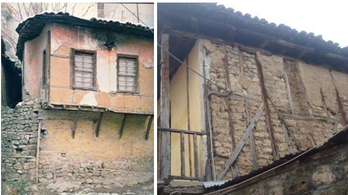
Fig. 12 Structural members of earth buildings
