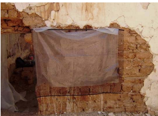
Fig. 24 Curing of grouted area
