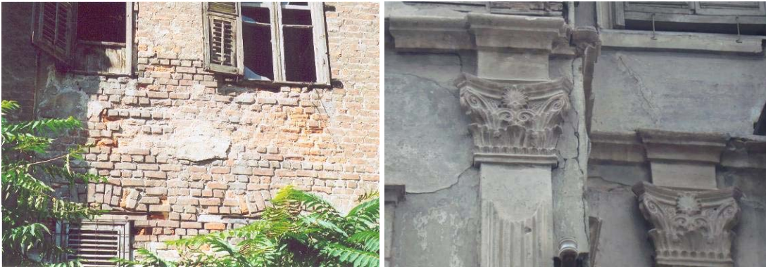
Fig. 6 Structural members of old building in Veria
