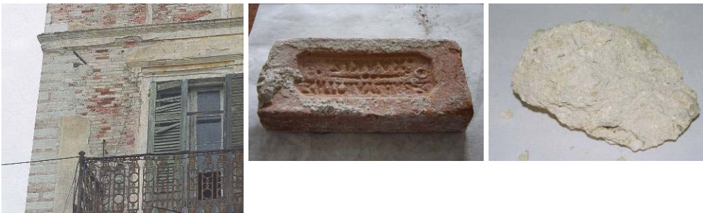
Fig. 9 Brick and mortar from an old building of eclectic architecture
