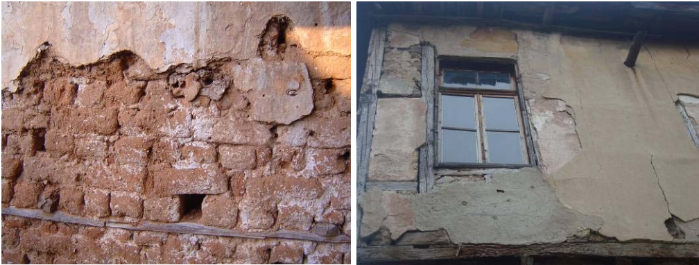
Fig. 14 Coverings of earth buildings
