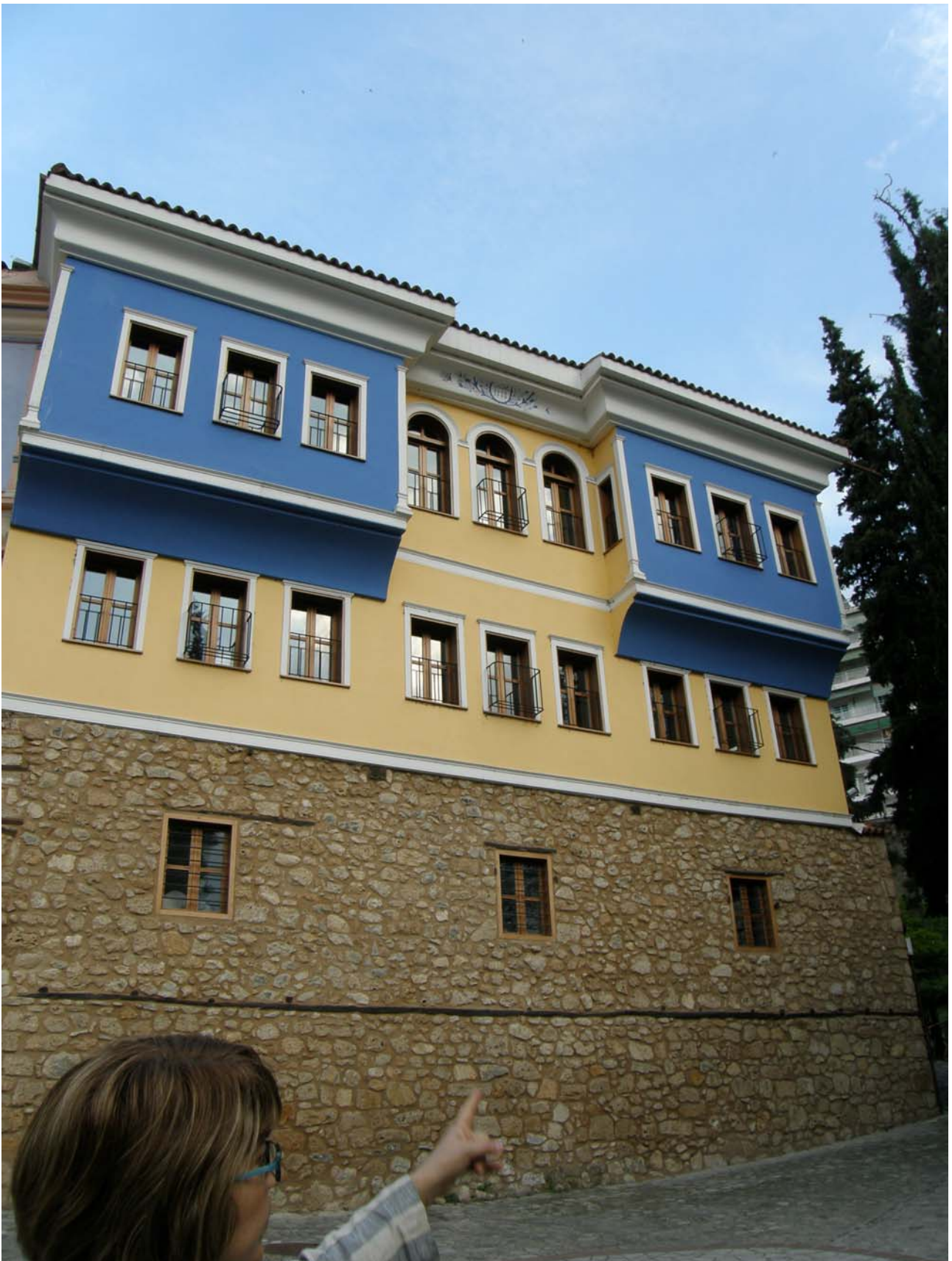
Figure 5: The same building after restoration.
