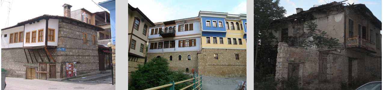
Typical traditional house of the historical city centre
