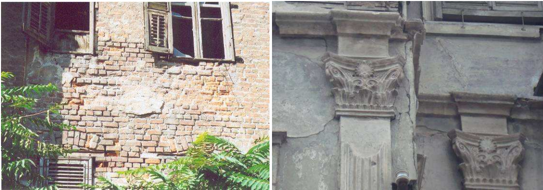
Fig. 6 Structural members of old building in Veria
