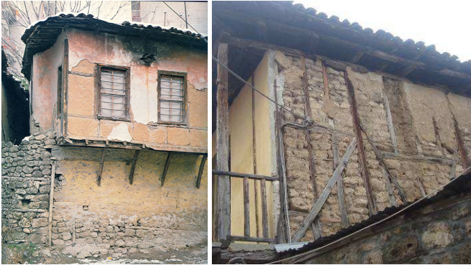
Fig. 12 Structural members of earth buildings
