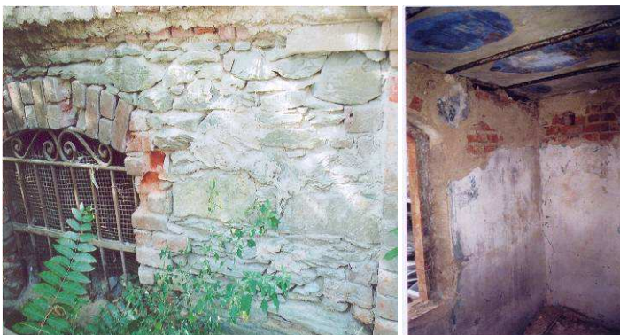
Fig. 5 Details of old structures in Veria
