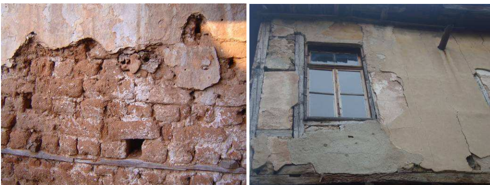
Fig. 14 Coverings of earth buildings
