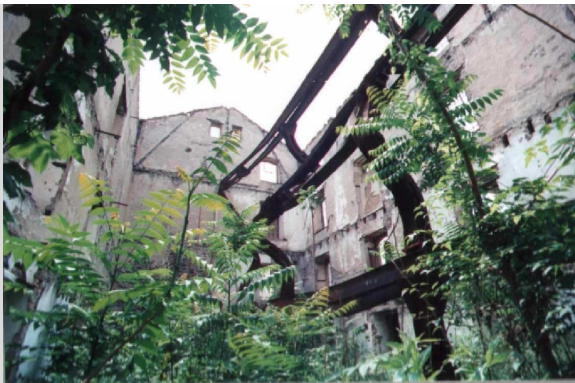
The internal space before the restoration works
