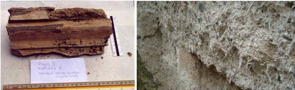
Fig. 10 Characteristics of materials of old neo-classic building
