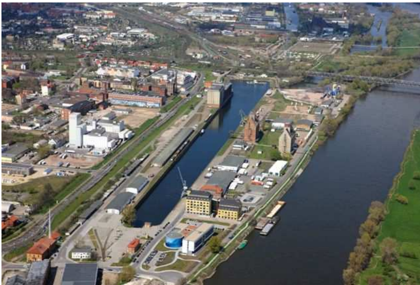
Figure 2. Aerial view of the Science Port, Magdeburg
