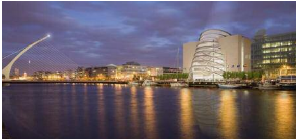
The Convention Centre (in figure a rendering of the project) will open in late 2010. It is one of the interventions which will promote tourism in Docklands
