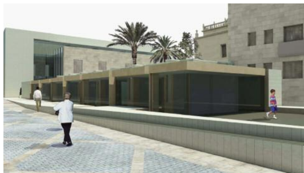
The image shows how the centre will be related to the public square and how will be recognizable in the urban texture
