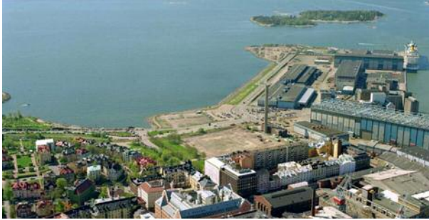
An over view of the future location of the cruise terminal
