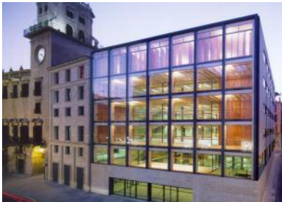
The enlargement of the 'Casa Consistorial': the main façade of the building
