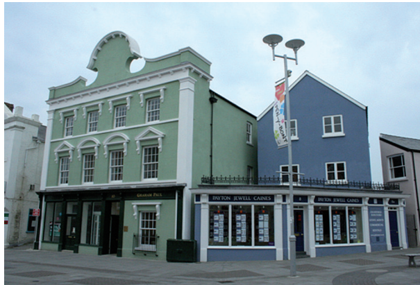
8-10 and 12 Durnaven Place, BTHIS with historical architectural details reinstated (Sash windows, slate roofs, stone detailing...), Bridgend, UK.
