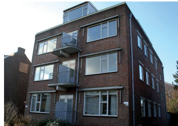
Social housing renovation with small scale CHP, Tuinwijk, Utrecht, Netherlands.
