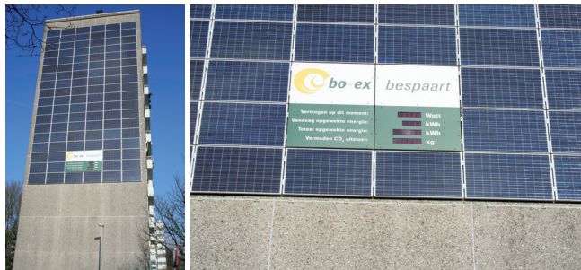
Solar water heating system, Utrecht, The Netherlands.
