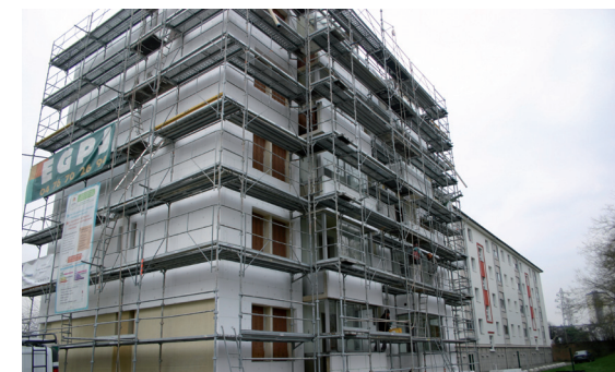
'La Bruyère' BBC level, renovation OPATB program, Echirolles, France.
