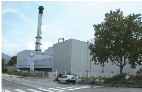
District heating Cie., Grenoble, France.
