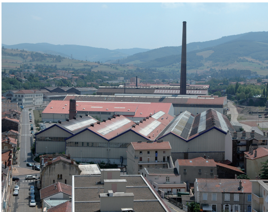
View of the GIAT Industry area in Saint-Chamond (© Epures)
