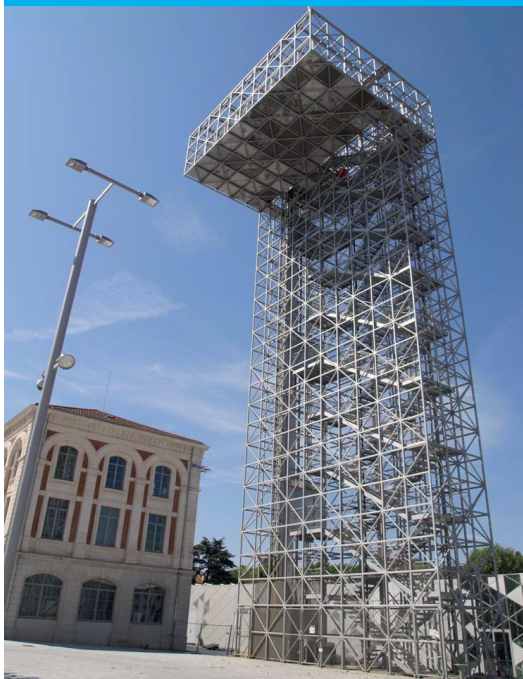
View of the GIAT Industry area in Saint-Chamond (© Epures)
