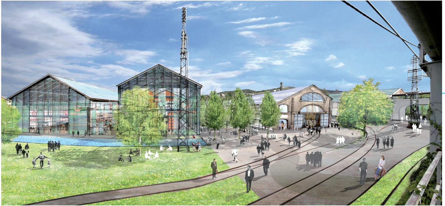
View of the GIAT Industry area in Saint-Chamond (© Epures)
