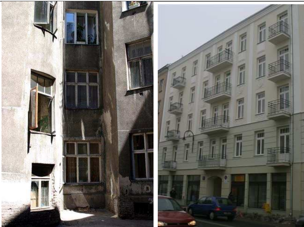
Ząbkowska Street 4 before and after repairs
