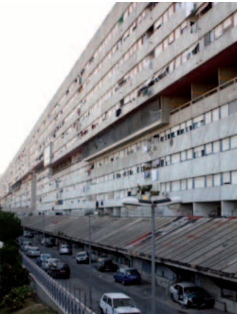
Figure 13. Corviale, the one-kilometer building in Rome's western outskirts
