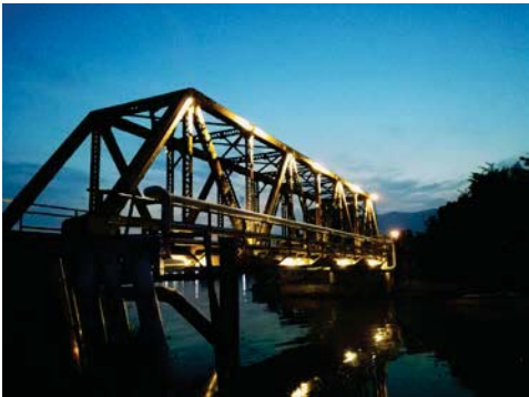
Illumination of the unused bridge
