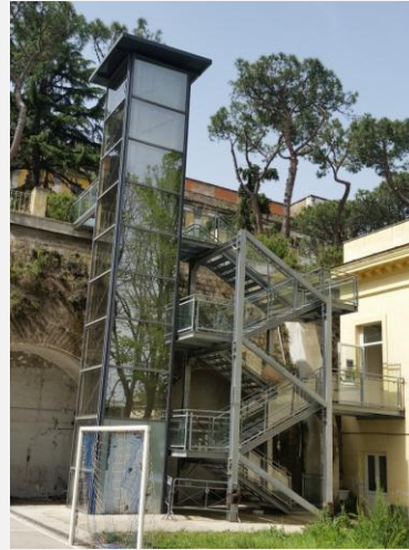
Staircase and elevator, connecting the internal gardens of the complex
