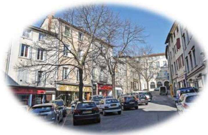
The place Perrot de Verdun before works
