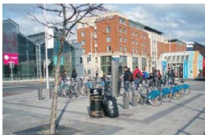
Dublin Bike Scheme, Custom House Quay. The retail development, CHQ building, and Jury's Inn, are visible in the background
