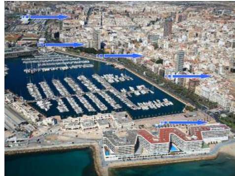
One of the goals is to find new ways to connect the port to the city centre and to combine the maritime activities with the ones located on the refurbished waterfront
