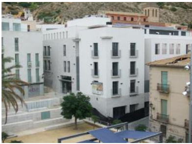
The building in the Plaza del Carmen will host 22 dwellings for students and a Social Centre ('Centro Civico')
