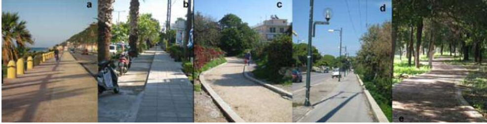
The pictures show various images of cycling paths built according the plan
