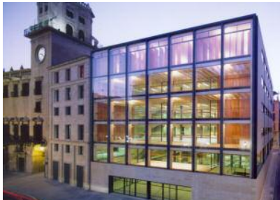
The enlargement of the 'Casa Consistorial': the main façade of the building
