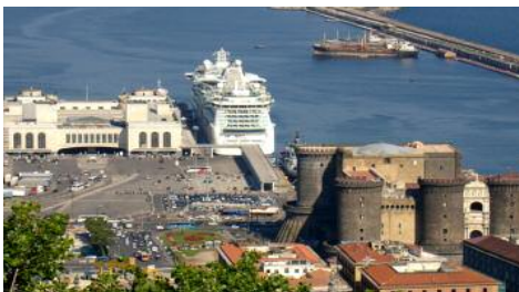
Naples Maritime Terminal, aerial view
