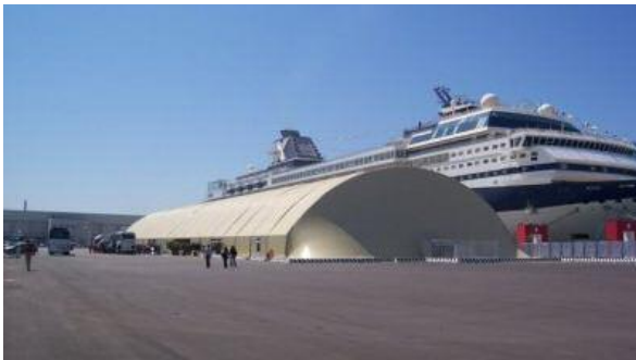
A temporary intervention for the terminal of Civitavecchia (Rome). (source: http://contex-t.ditf-denkendorf.de/ )
